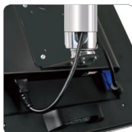
Neatly installed cables
